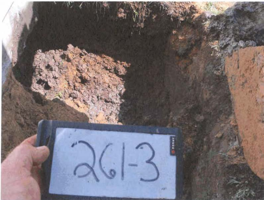
Picture 4: UST 261Beech-3 excavation.
