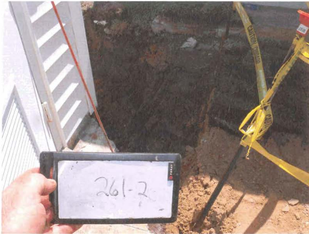
Picture 3: UST 261Beech-2 excavation.
